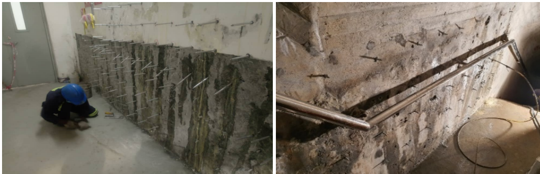
Figure 6: Curtain grouting at EL1037 and stairs to EL1017
