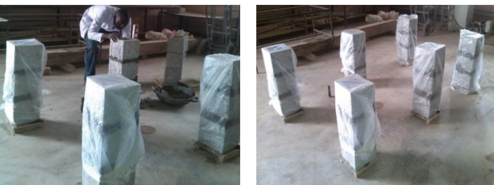
Figure 2: Construction of Masonry Hollow Concrete Block Prism Column
