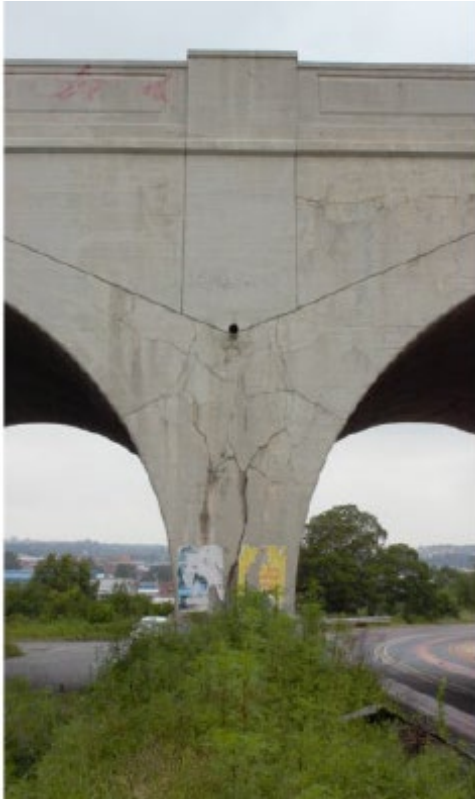
Fig. 5, 6, 7, 8 : Evidence of map-cracking on various bridge elements
