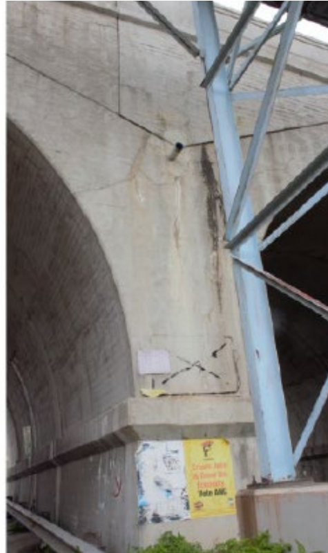
Fig. 5, 6, 7, 8 : Evidence of map-cracking on various bridge elements
