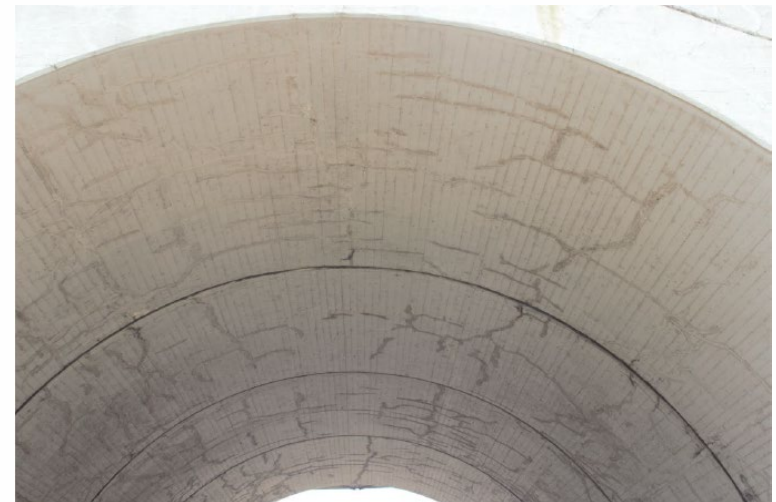
Fig. 5, 6, 7, 8 : Evidence of map-cracking on various bridge elements
