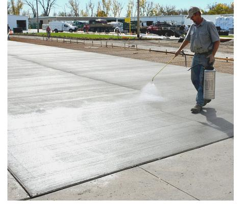
Concrete that has been correctly specified, batched, mixed, placed, and finished can still fail without adequate curing. "Curing is usually the last step in a concrete project and, unfortunately, is often neglected - even by professionals," says Bryan Perrie, CEO of Cement & Concrete SA (CCSA).
