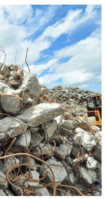
Crushed concrete furthermore absorbs carbon dioxide. Precast components from structures can be reused in new buildings without having to be demolished and recycled. Structures using precast elements should, in fact, be designed for such reuse.
