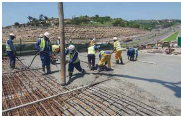
Photo 6: Ramp A1 Cast In-situ Deck
