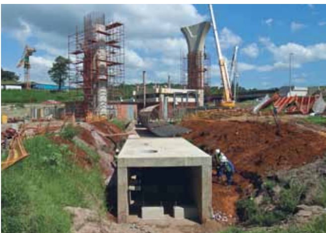
Photo 9: L-R: Services and Stormwater Culverts
