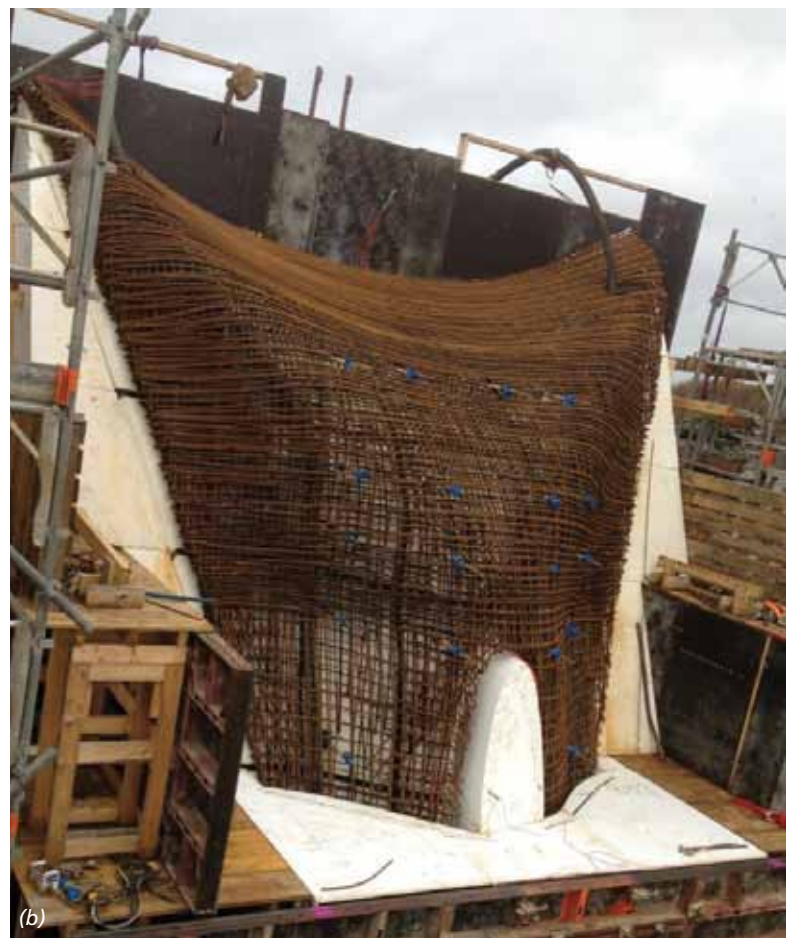
Fig. 7: Initial work at the construction site: (a) the assembled first layer of formwork; and (b) steel reinforcement. A complete 3-D model of the reinforcement was developed, and the more complex bars were fabricated using robots. However, most bars were designed to be fabricated conventionally using standard machinery
