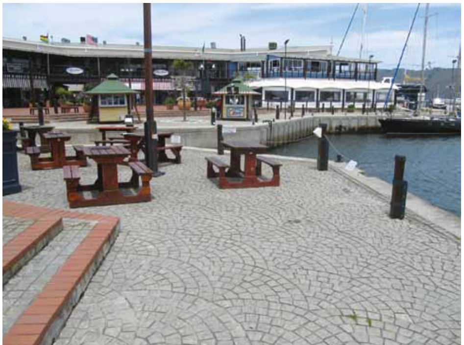
Fan cobble paving blocks at Knysna Waterfront by Smartstone
