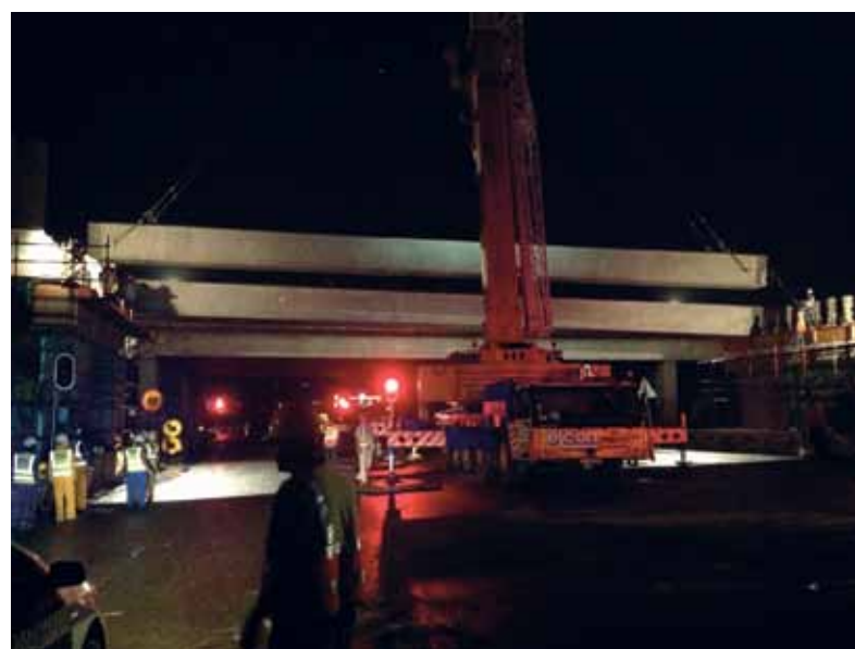
Photo 3: Placement of the precast beams at night
