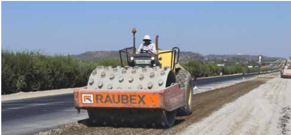
Raubex is stabilising the sub-base to a depth of 350 mm with AfriSam's Roadstab 32.5N CEM ii B-L cement.
