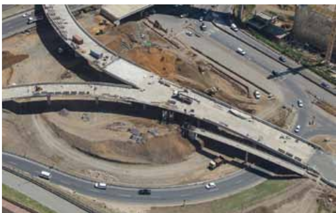
Photo 4: Ramp D2 Bridge Voided Deck
