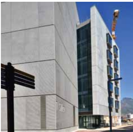
No 1 Silo 3: Precast panelling at No 1 Silo by Concrete Units
