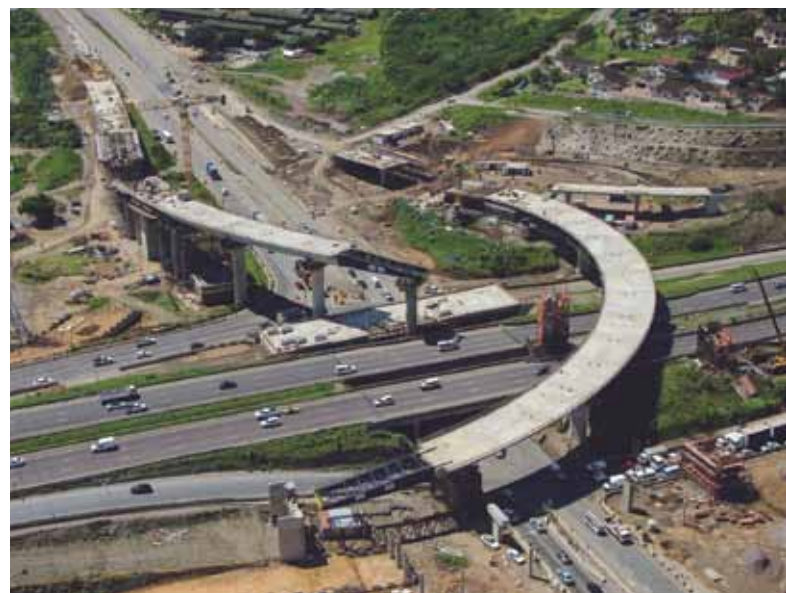
Photo 2: Ramp D1 Incremental Launch Bridge 106m Radius of Inclined Circle Launch Path
