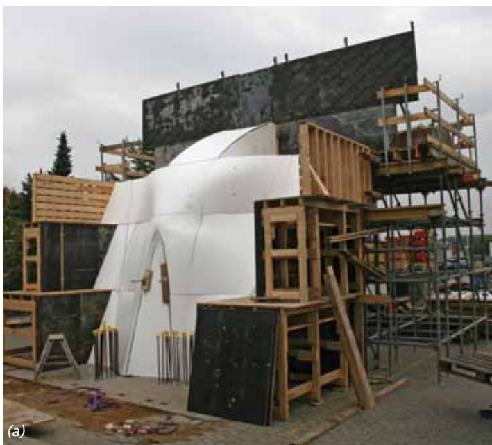
Fig. 7: Initial work at the construction site: (a) the assembled first layer of formwork; and (b) steel reinforcement. A complete 3-D model of the reinforcement was developed, and the more complex bars were fabricated using robots. However, most bars were designed to be fabricated conventionally using standard machinery
