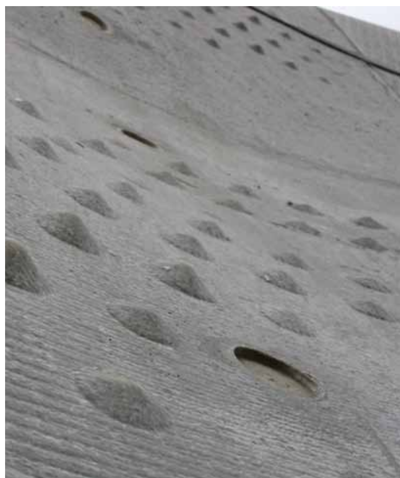
Fig. 9: A close view of the surface of the Demonstrator reveals the extra detailing applied in the milling process
