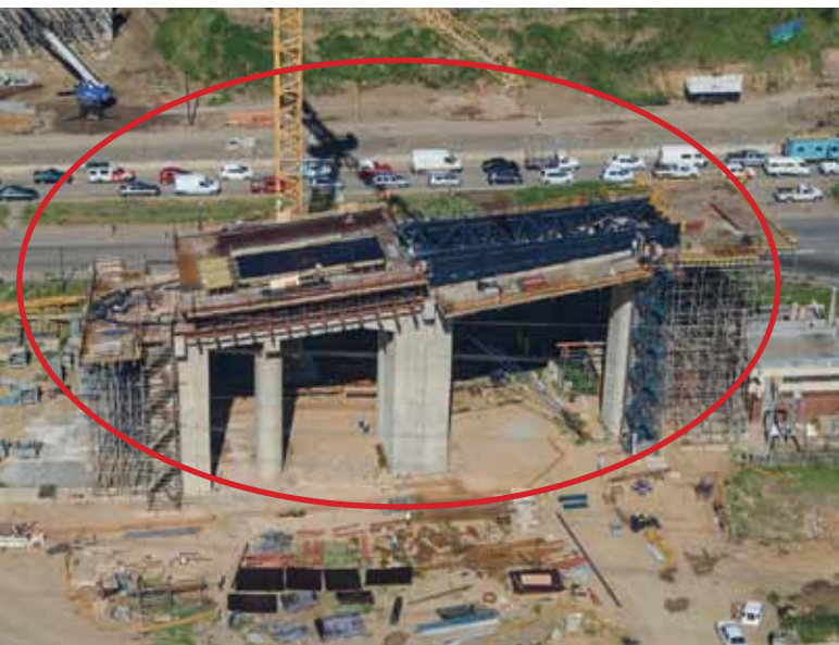
Photo 1: Ramp A1 Incremental Launch Bridge Elevated Casting Yard
