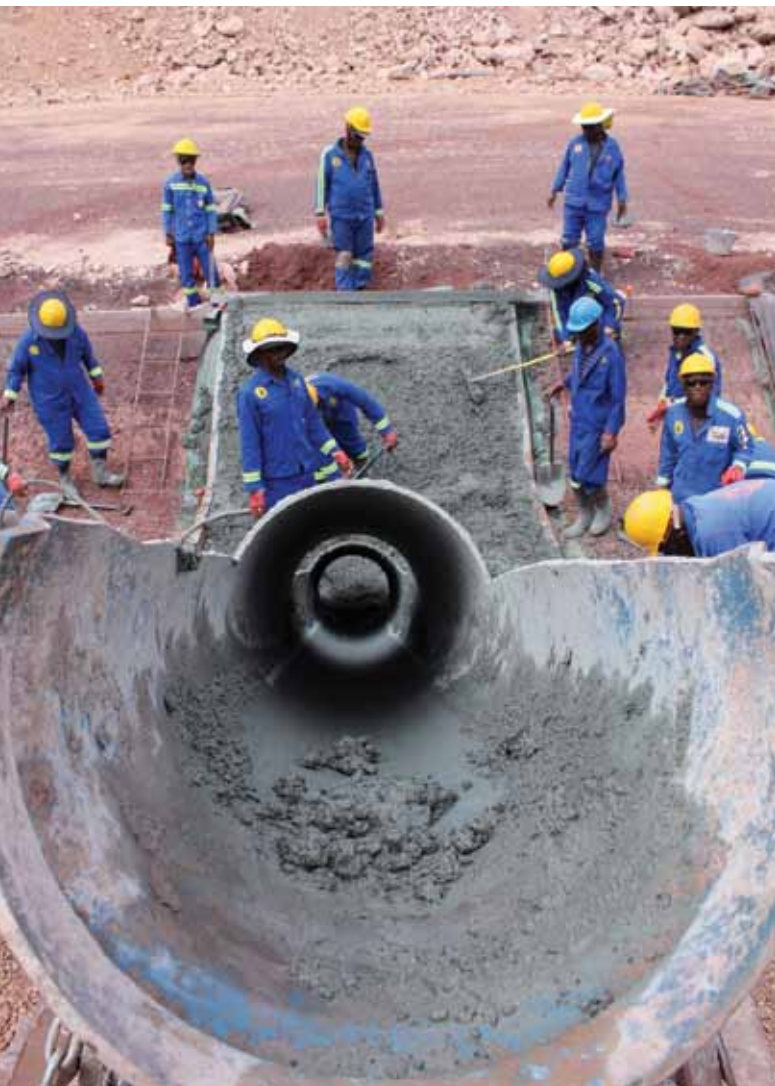
A novel chute system has allowed the contractor to do away with a mobile crane and boost productivity.
