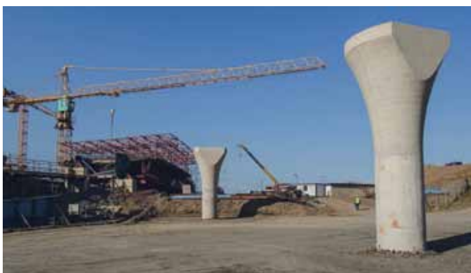
Photo 5: Ramp D2 Bridge “Shaved Golf Tee” Shaped Piers
