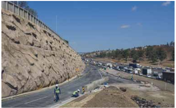
Photo 8: L-R: Mechanically Stabilised Earth Wall and Rock Anchored Sprayed Concrete Wall
