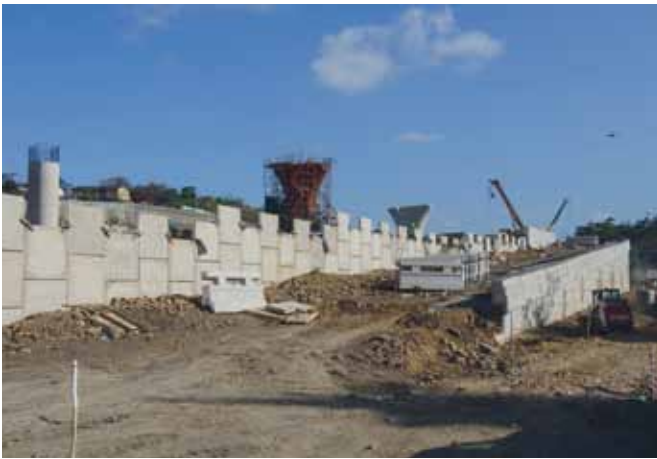
Photo 8: L-R: Mechanically Stabilised Earth Wall and Rock Anchored Sprayed Concrete Wall
