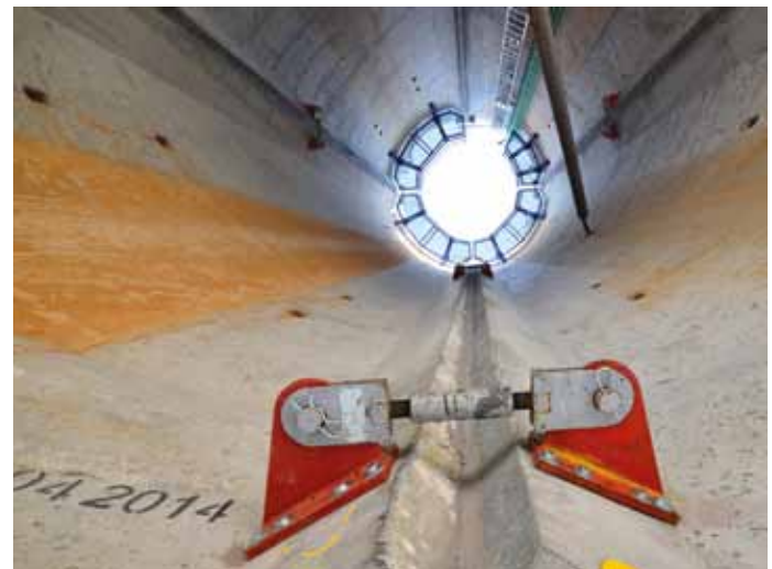
Internal view of a T1 section showing the bowtie joint.
