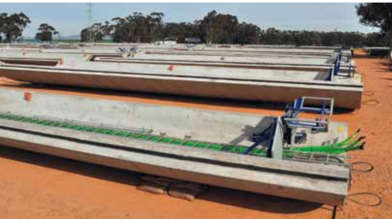
Concrete segments prior to assembly.
