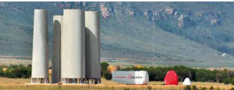
Tower segments stacked together prior to assembly.
