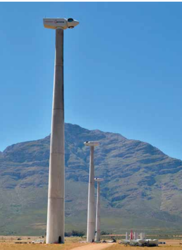
Some fully assembled precast concrete towers.
