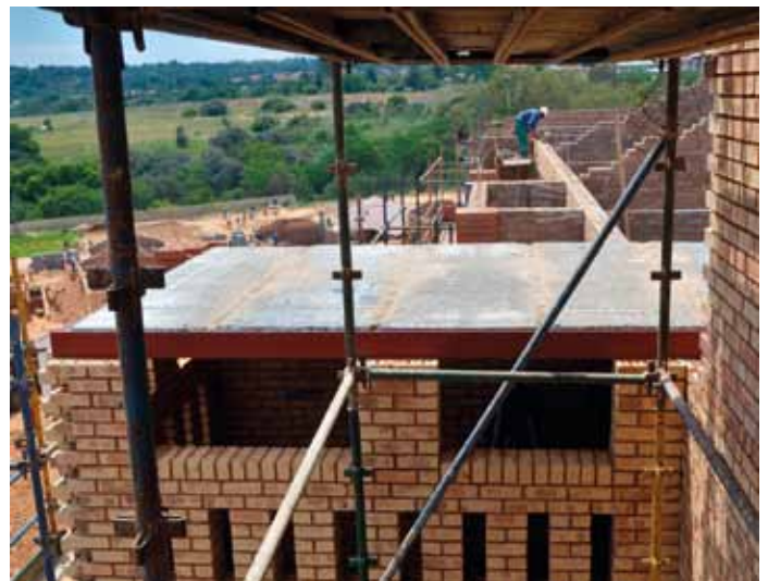
Reinforced slab installation at Olivedale Retirement Village.
