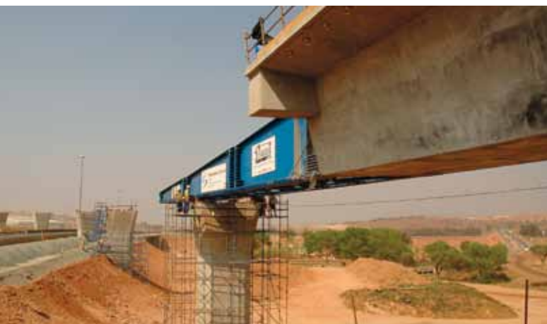
Launching the switch ramp onto coffin-shaped piers
