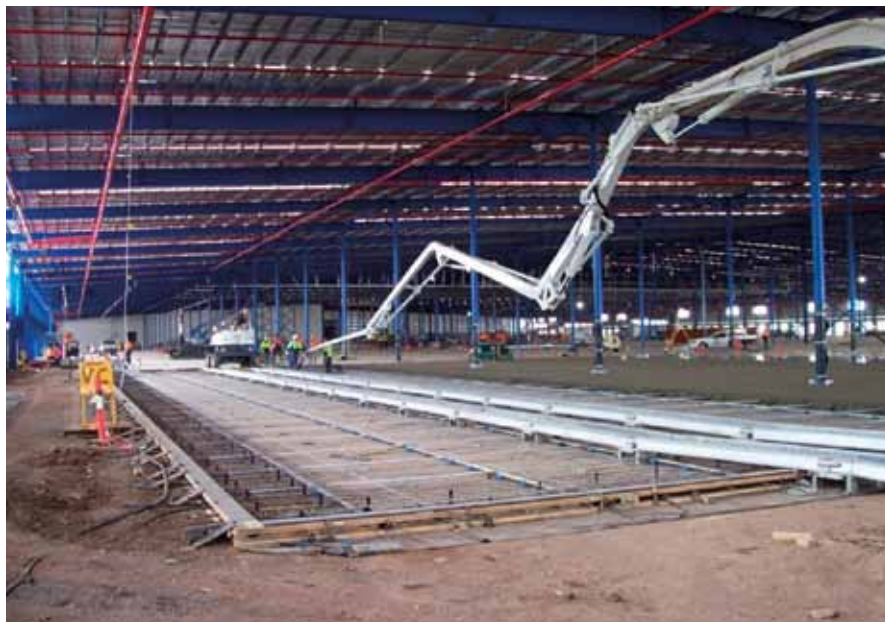
Pumping concrete for post-tensioned floor.
