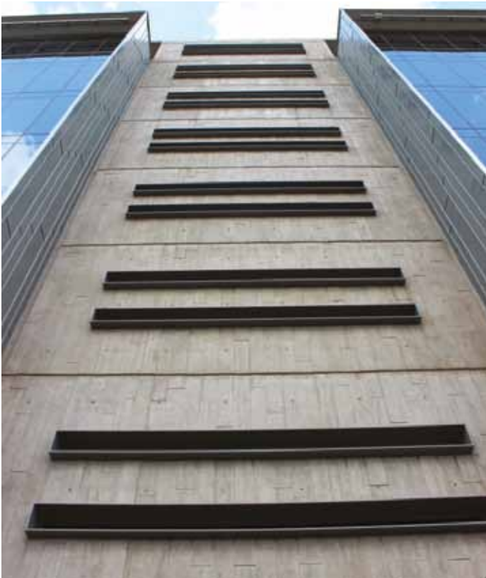
South façade, concrete walls with timber grained off-shutter textured finish.
