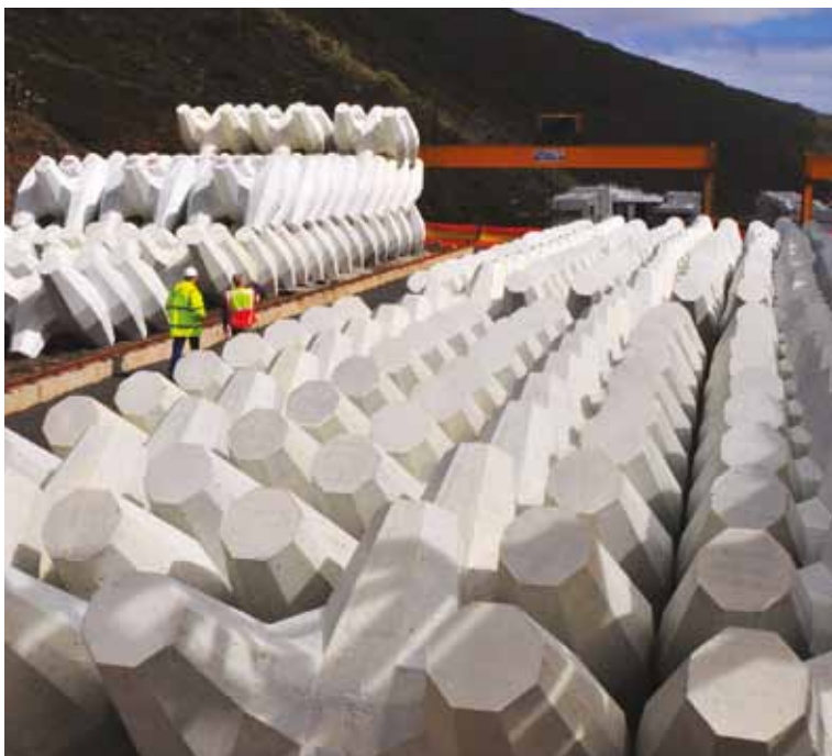
Over 700 units of precast Core-loc armour units (7 tonnes per unit) and hollow blocks (27 tonnes per unit before filled with stone) were placed by crawler cranes via GPS around the wharf from the surface bed to just above sea level.
