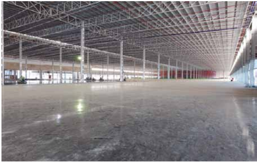
How exactly, would you assess level and flatness characteristics of this floor with a straight-edge?
