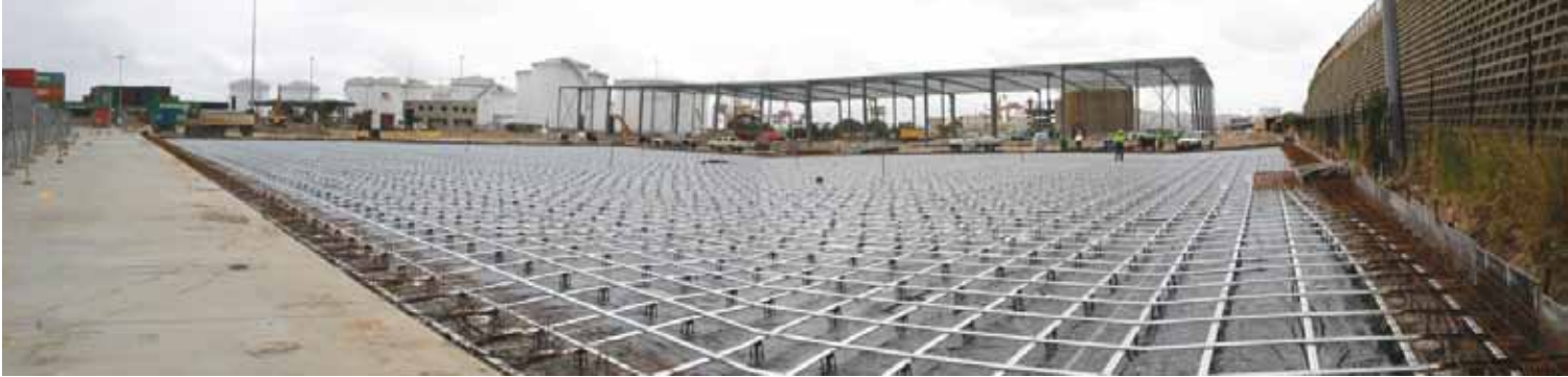
External slab prior to pour with bonded PT
