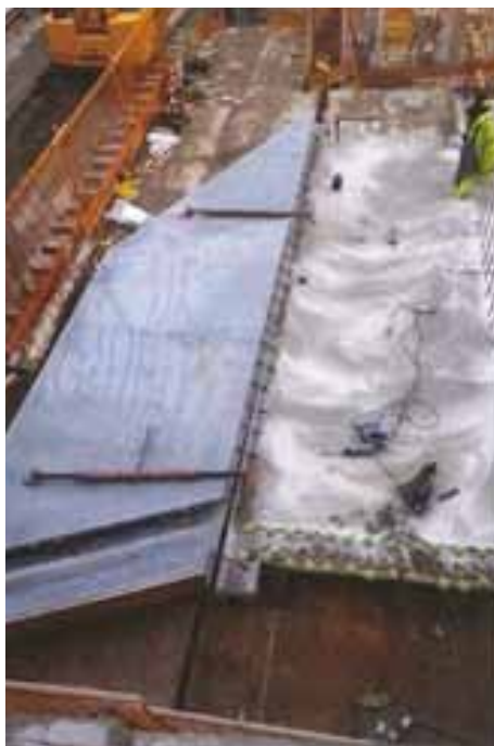
Concrete twin wall systems are hybrid in-situ/ precast building products used to construct concrete walls quickly. The product comprises of two leaves of reinforced concrete held apart by reinforcement lattices.
