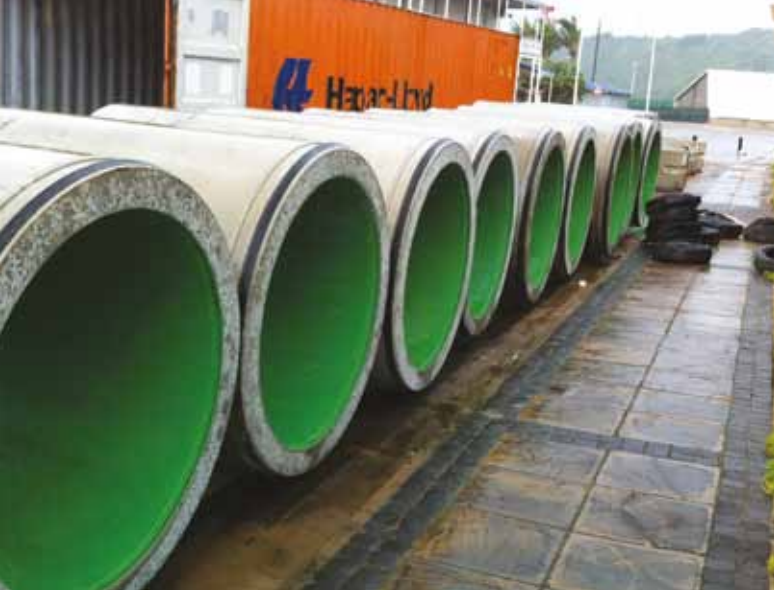
Stack of pipes awaiting jacking.
