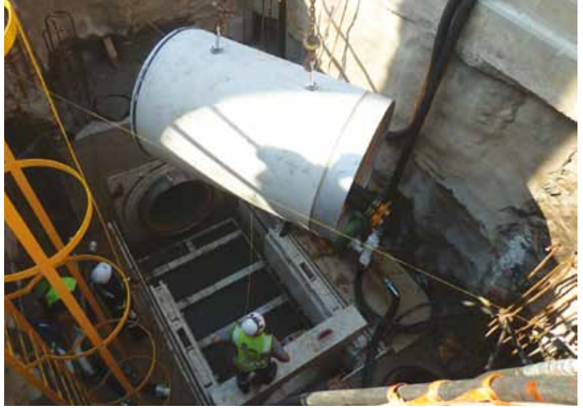
Pipe section being lowered into jacking pit.
