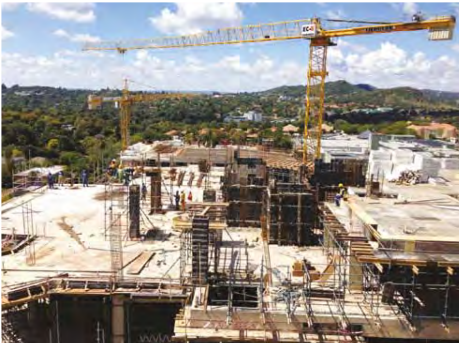
Construction makes use of conventional concrete reinforced slabs. Phase 3 is located at the lowest level of the Lynnwood Bridge complex in terms of elevation, necessitating lateral support being incorporated to anchor the complex.
