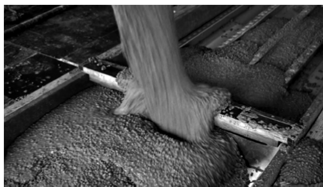
Figure 6. Casting a composite slab with pumped SCLC.
