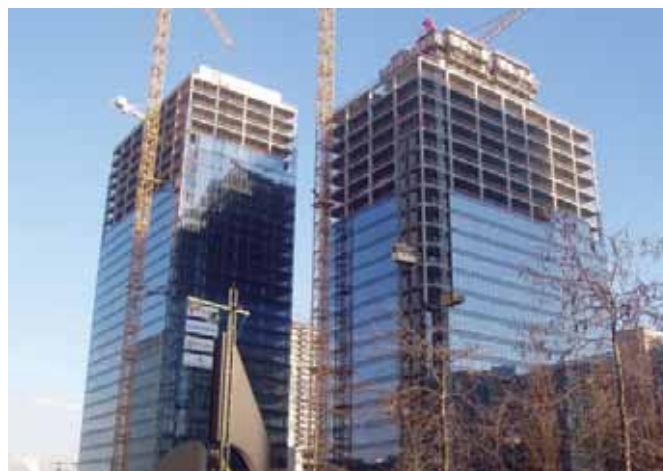
A precast frame structure (columns, beams, slabs, shear walls) in Europe (Arnold van Acker, Belgium).
