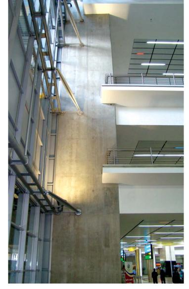
large spans, limited structural depth and high permanent loads on the slabs. The huge oval atrium of approximately 50 m x 40 m above the central concourse area on the arrivals levels is the focal feature.
