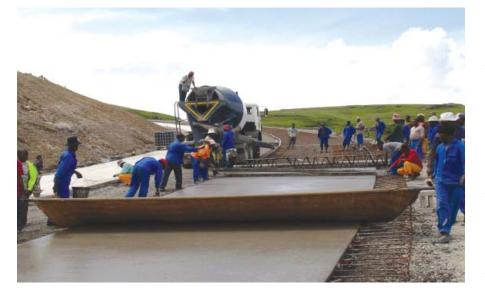
er in the tertiary crushing phase. Several trial mixes were designed and tested on trial sections of concrete pavement. The mix designs were modified according to workability criteria, and strengths were verified by laboratory control testing. A higher cement content than the minimum specified cementitious content of 265 kg/m<sup>3</sup> had to be used in order to achieve a more workable mix. This was despite the addition of a plasticising admixture.
