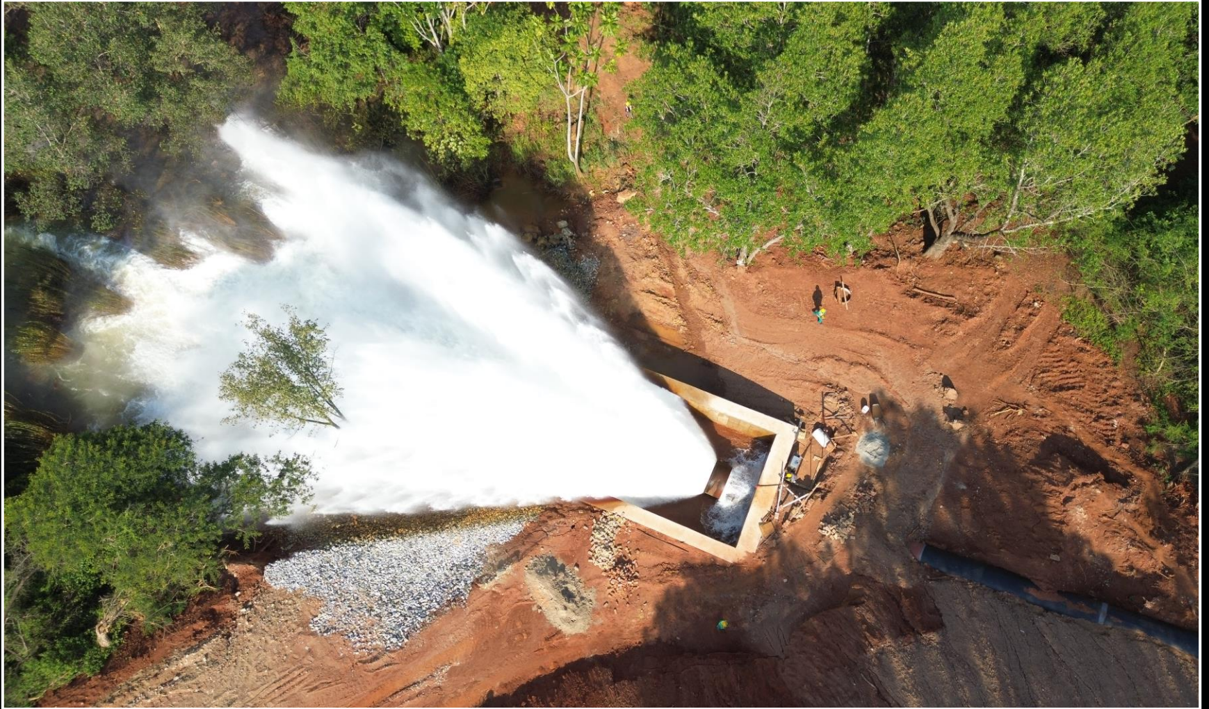
River Diversion Outlet
