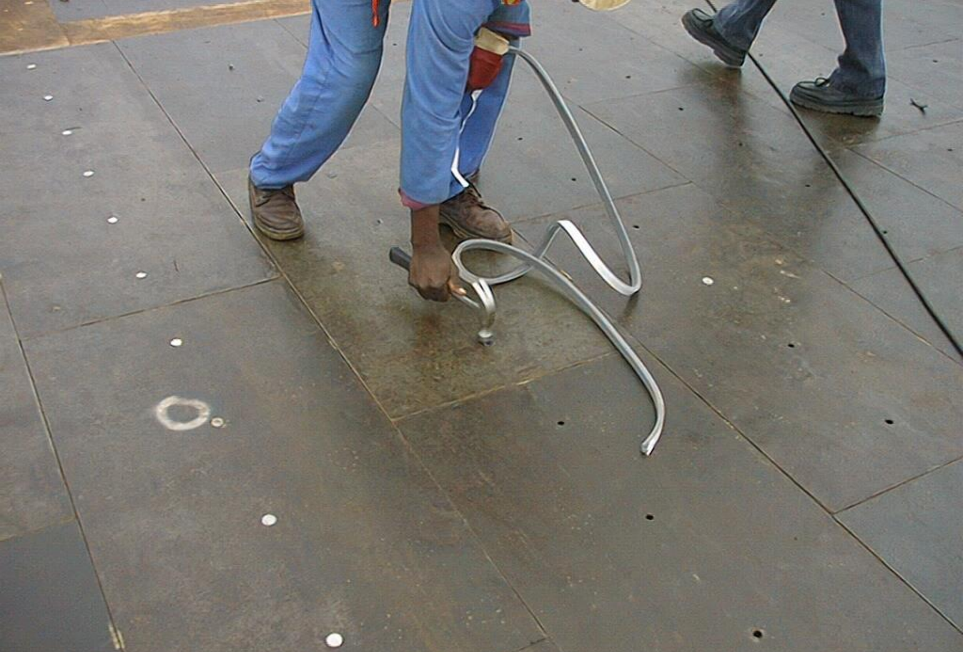
Self-adhesive compressible foam gaskets provide an excellent seal against grout loss.
