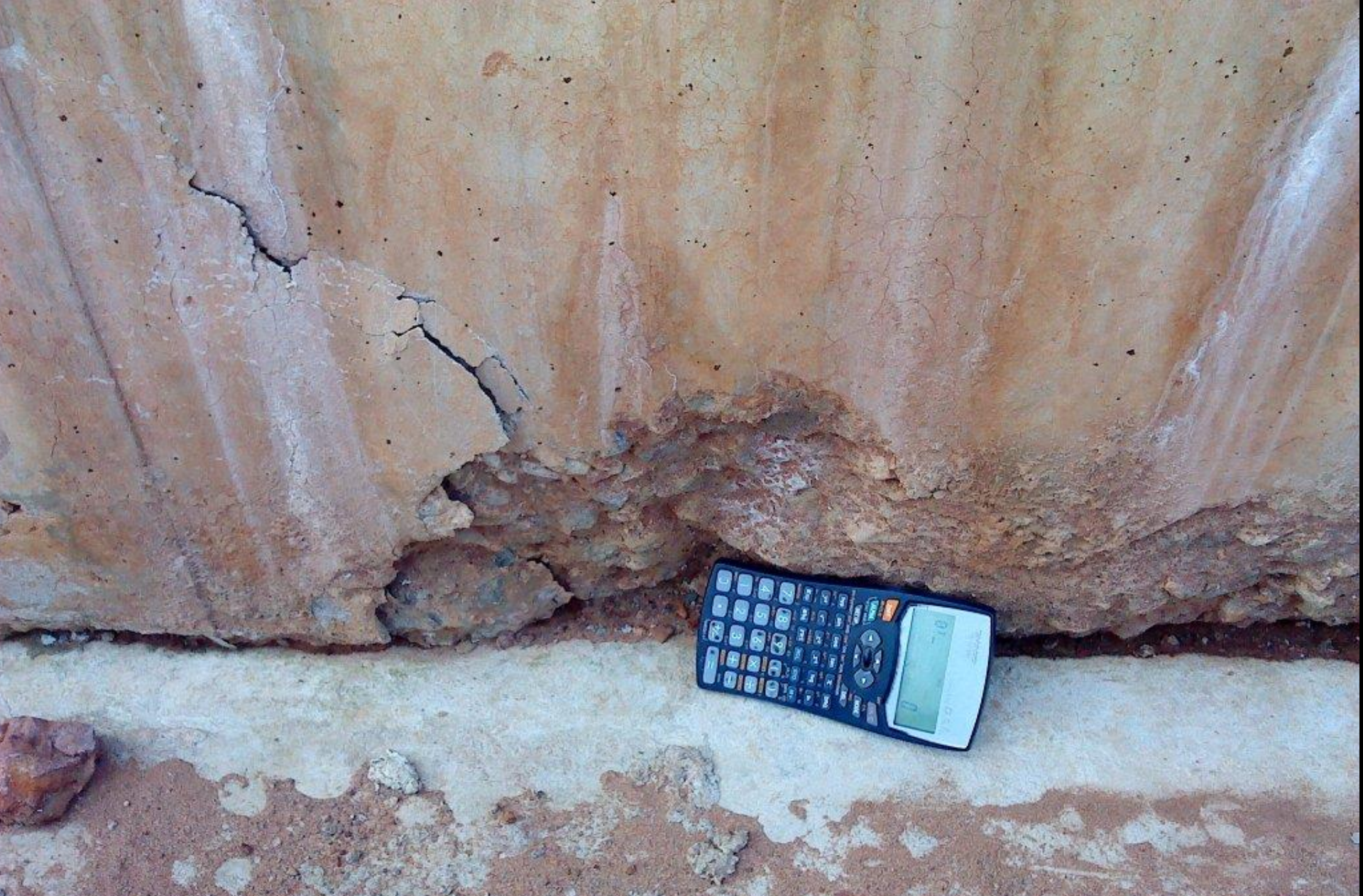
Cylindrical wall founded on a Kilcher type rubber/PTFE bearing with bandage seal between wall and floor on inside.
