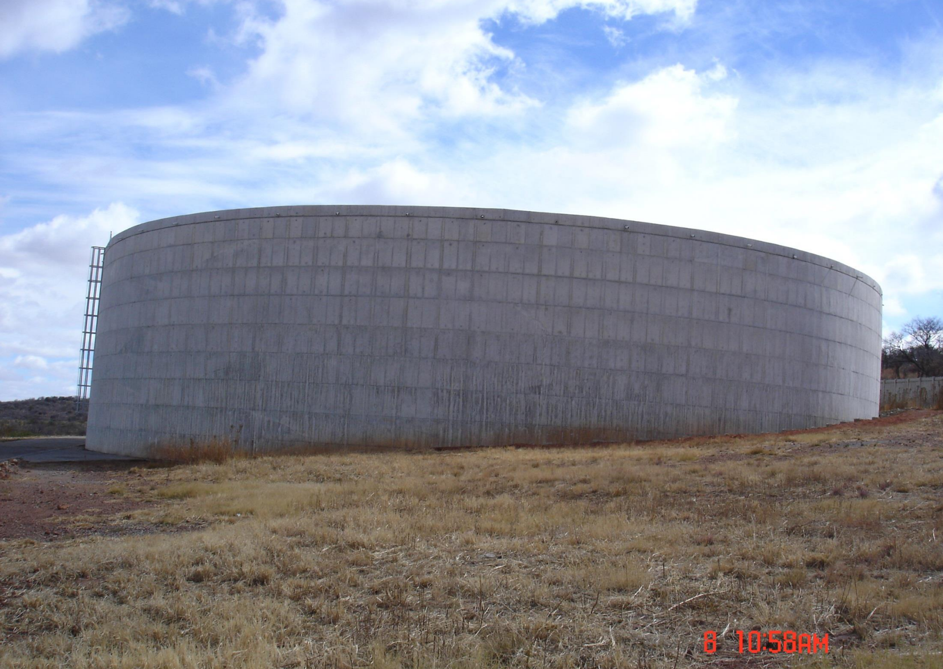
After a few weeks of autogenous healing – no leakage.
