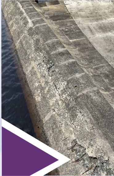
Reinforcement corrosion
